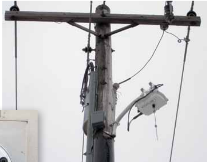
The router, pictured on the pole above, receives usage information from the new Gridstream meters (left).
