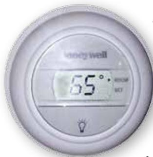
The newer Honeywell thermostats are now digital and require additional electricity, but they get it from the control on the burner and not from batteries. (It is not possible to use this type of thermostat with all oil burner controls because some of them do not have a transformer for sending voltage back to the thermostat.)
