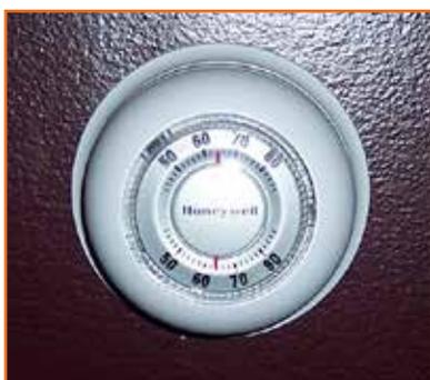
models. The old models worked by turning the dial which causes mercury in a tube to make a connection between the two wires and activate the furnace. Simple system with no extra frills that require no additional electricity.
