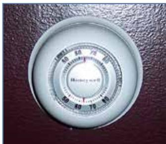
old models worked by turning the dial which causes mercury in a tube to make a connection between the two wires and activate the furnace. Simple system with no extra frills that require no additional electricity.
