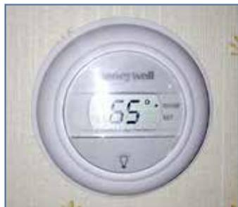
The newer Honeywell thermostats are now digital and typically require additional electricity but they get it from the furnace fan center and not from batteries.
