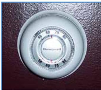
batteries whether they are the older gold models or the newer white models. The old models worked by turning the dial which causes mercury in a tube to make a connection between the two wires and activate the burner. Simple system with no extra frills that require no additional electricity.
